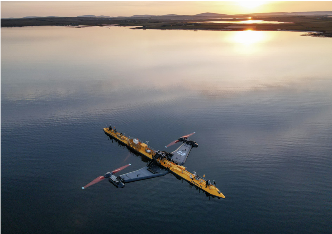
Aerial shot of O2 turbine off the Orkney coast. © Orbital Marine Power
