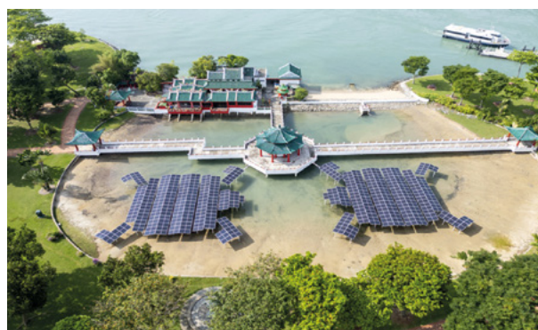
Figure 8: Renewable system deployed in Kusu Island, Singapore to meet the energy needs of the island
