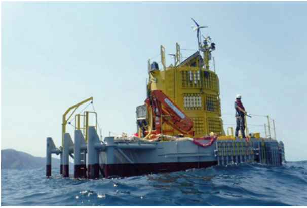
HarshLab installed at BiMEP
