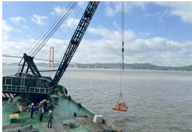
Deployment of test equipment in Zhoushan test site
